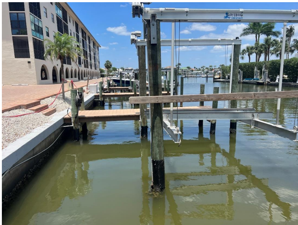
Photo 1: View of seawall, docks, and waterway looking northeast.
